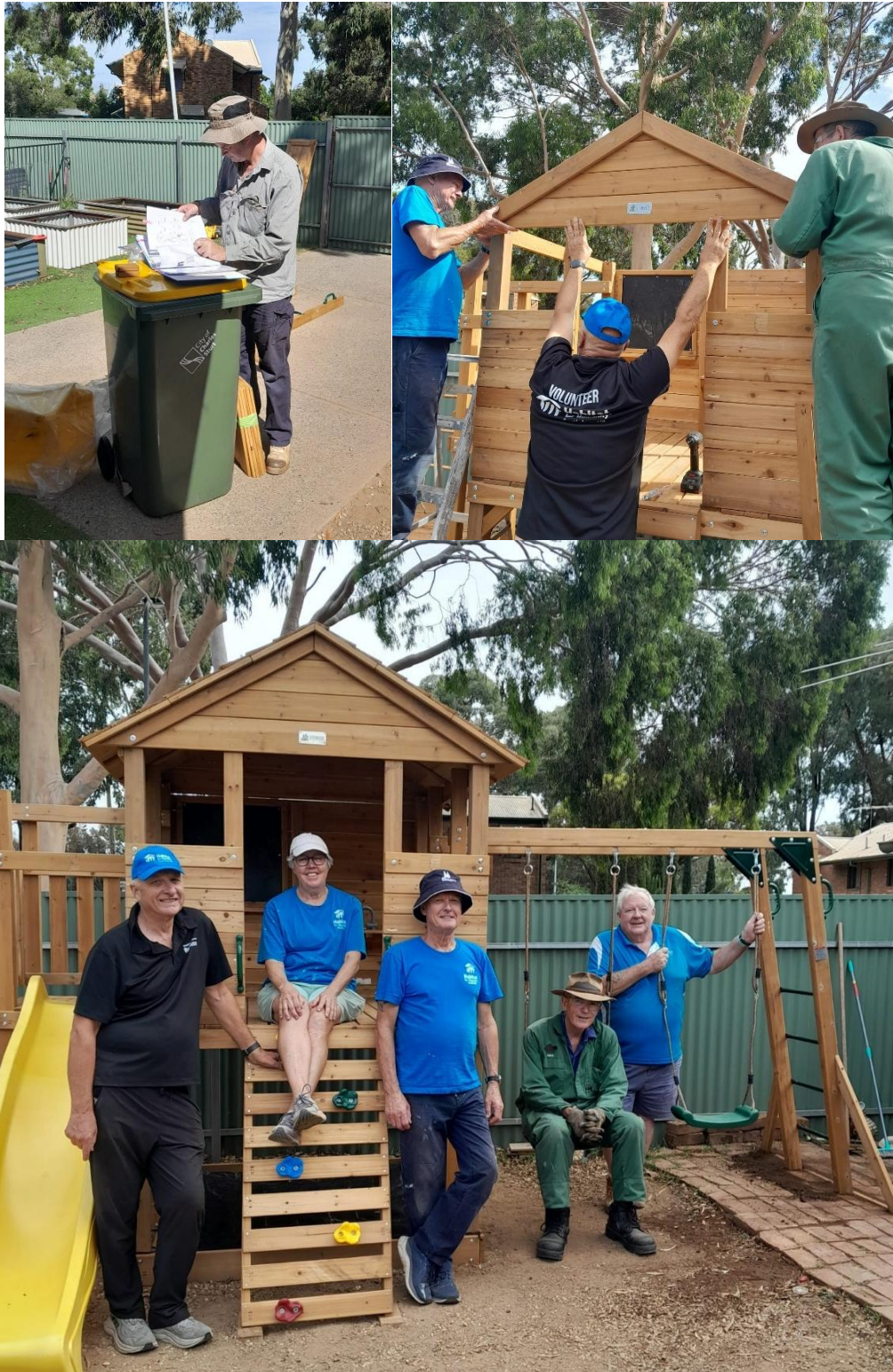
Building a cubby house for a kinship carer involved 31 hours of volunteer labour.
